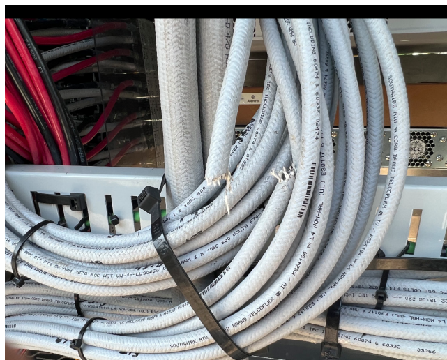
Left: Successful cuts and theft of wire in equipment cabinet. Top right: Cuts to wires on utility pole in conduit. Bottom right: Cuts to wires on utility pole in cabinet.
